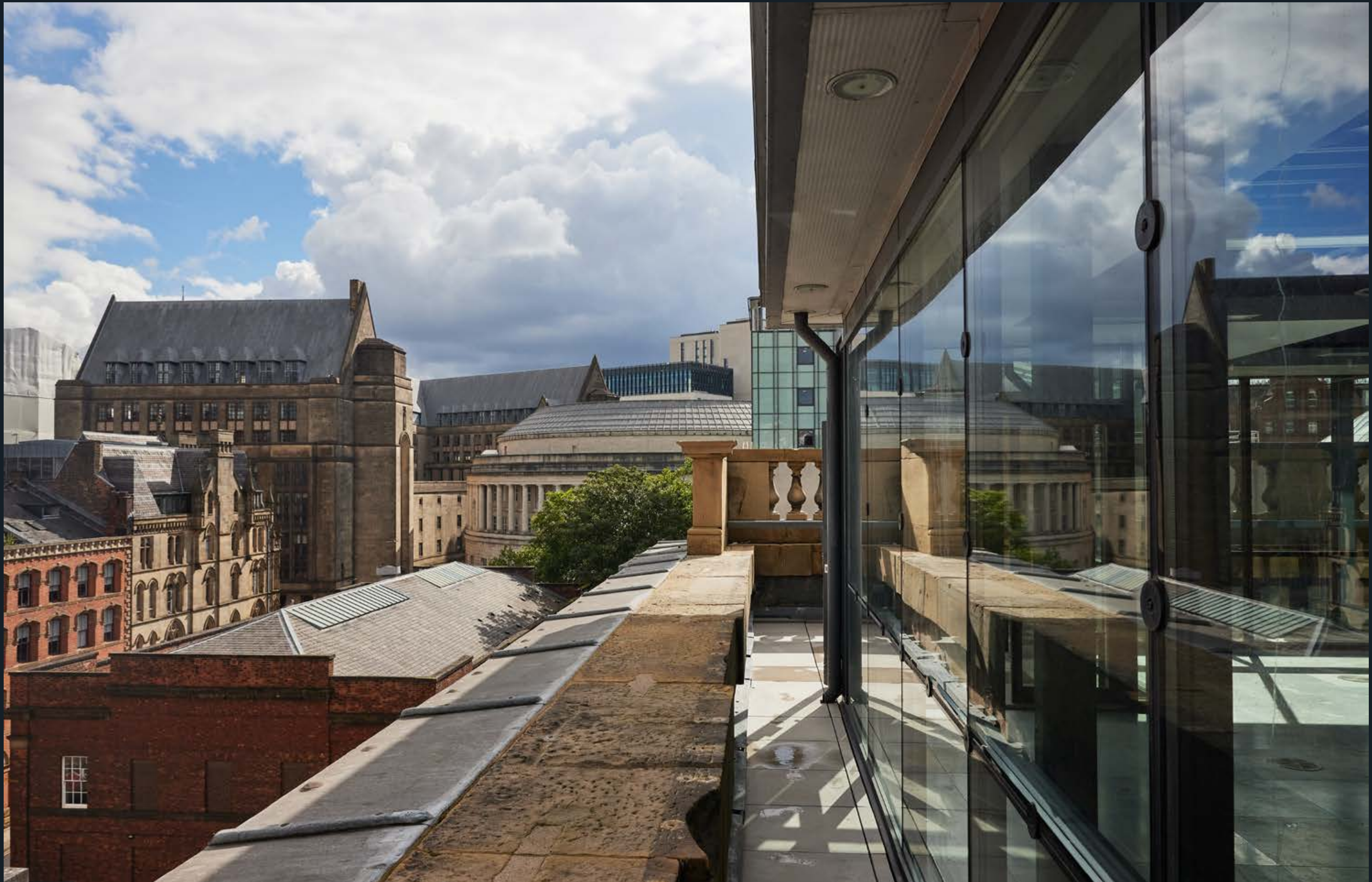
— Impressive views of Manchester Central Library and the town hall
